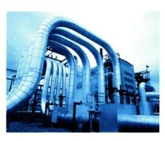
the state of the insulation. "The condition of the insulation and top cover conditions are the key points to determine how long the inhibitor will last," he says, adding that inhibitor can be applied either manually or with an automatic injection system.
